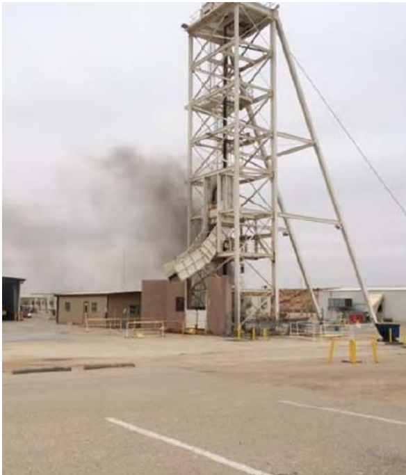
Figure D-36. Smoke exiting the salt shaft ee
